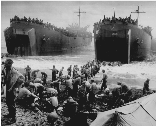
Two Coast Guard-manned LST's open their great jaws in the surf that washes on Leyte Island beach, as soldiers strip down and build sand-bag piers out to the ramps to speed up unloading operations. - 1944.
